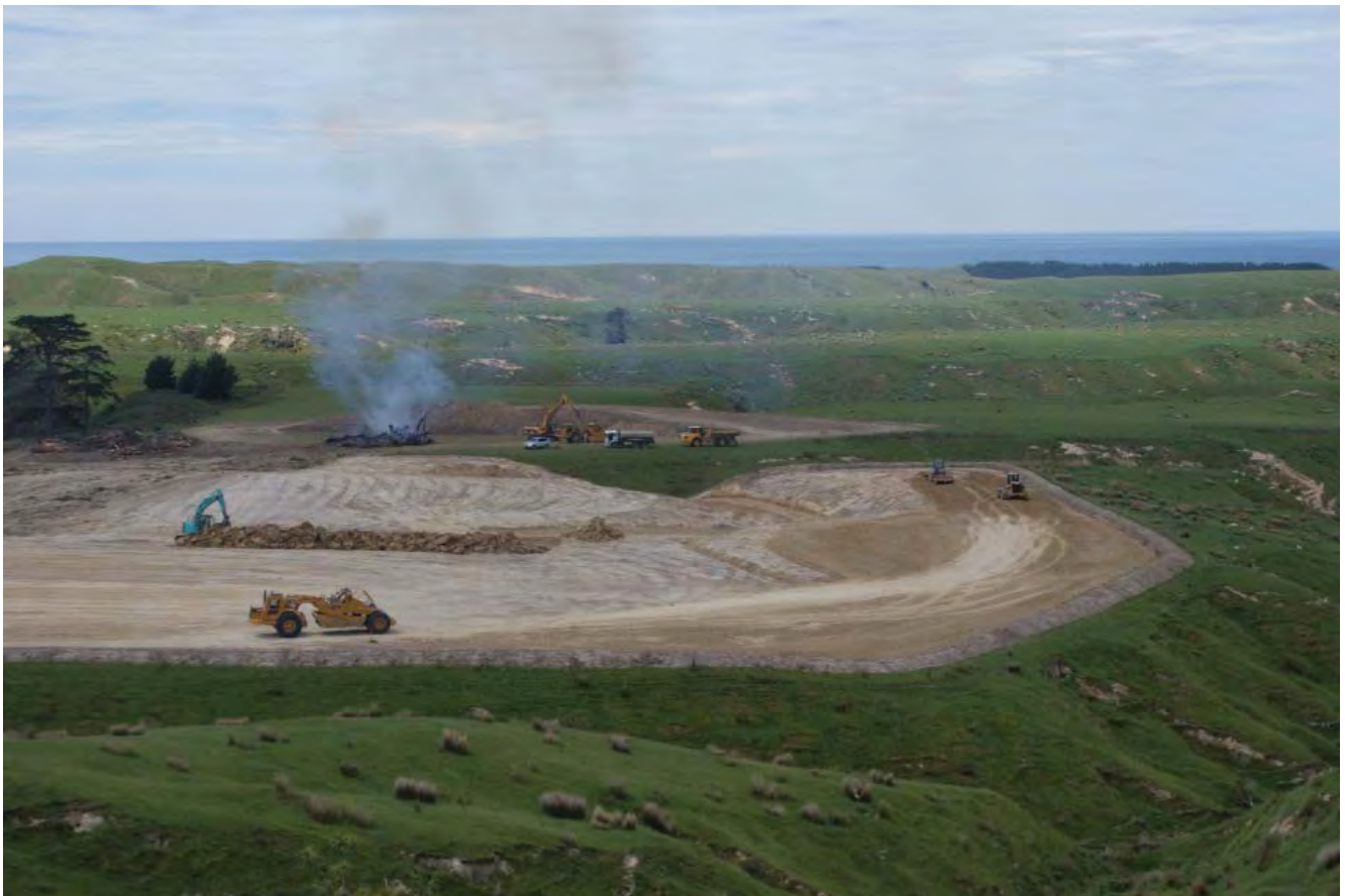
Earthworks at the new Riversdale Beach Sewerage Scheme.
