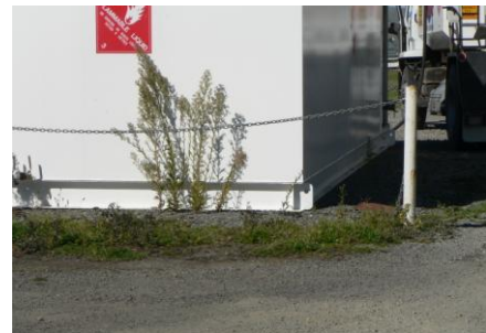
Weeds requiring maintenance (Issue: aesthetics and weed propagation)
