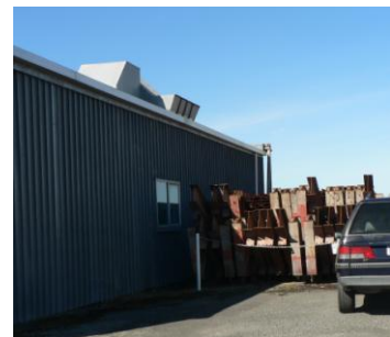
Example of roof services requiring specific design (colour and location). Note unacceptable storage alongside building)
