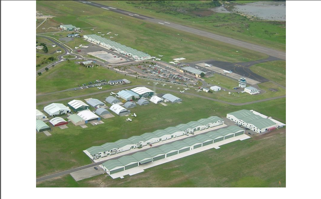
Example multi-hangar development in foreground: Tauranga
