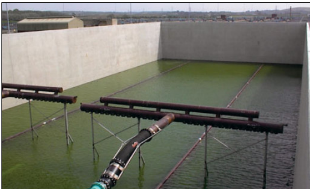
Figure 5-2: Inside a Continuously Fed SBR
