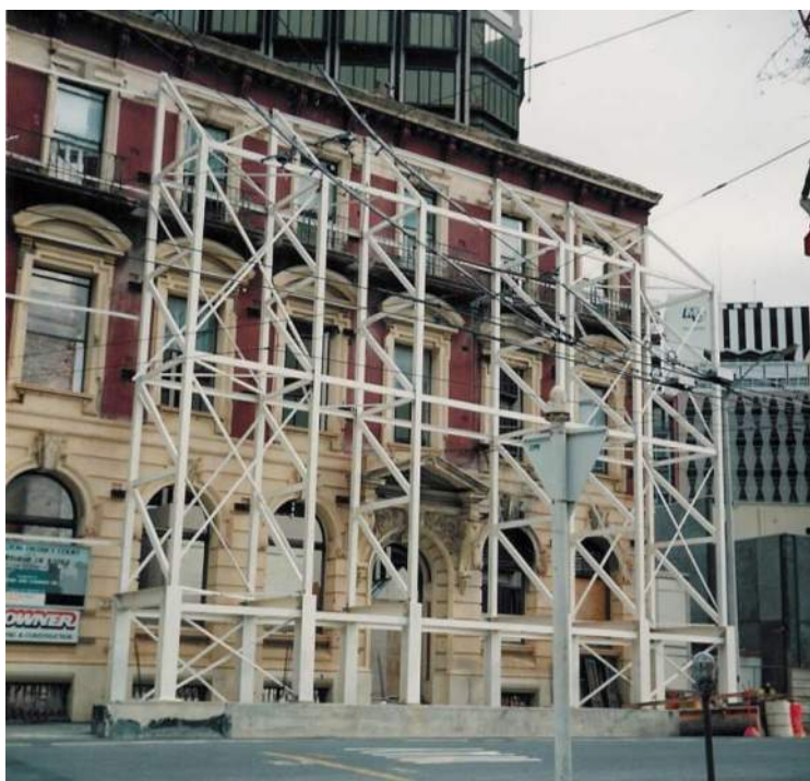
Figure 3.5 - Example of Façade Retention Temporary Works (Wellington District Court)
