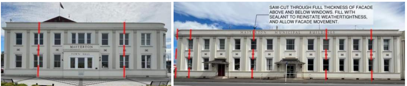
Figure 3.4 - Possible Intervention to Destiffen Façade
