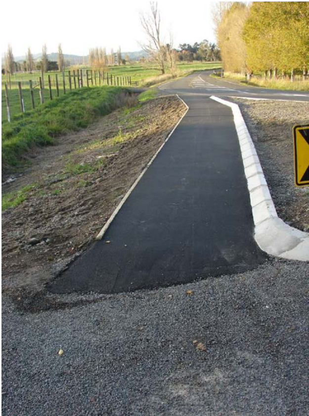
Lees Pakaraka Road is on a popular sports cyclist training circuit. This short stretch of cycle path enables cyclists using the circuit to more easily merge with traffic on Masterton-Stronvar Road
