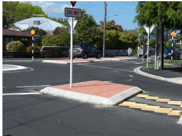
This improvement of the Renall Street/ Pownall Street intersection slows all traffic through adding a very small roundabout, kerb build-out areas, and median waiting areas for crossing pedestrians. It helps both pedestrians and cyclists, and improves overall road safety.
