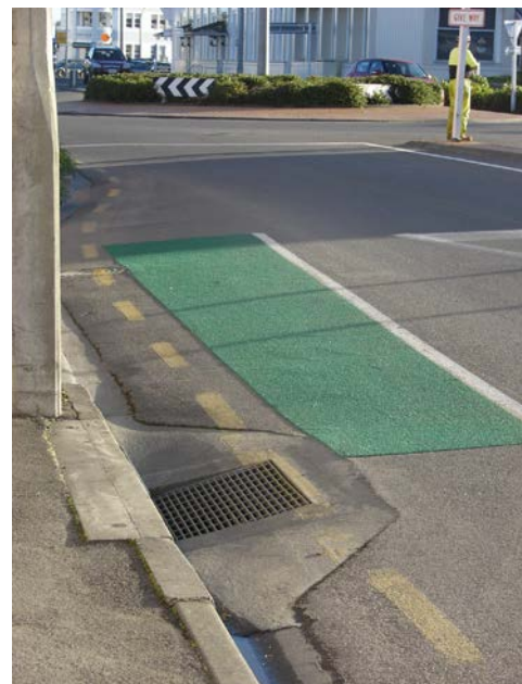
Green surfacing to alert motorists to cyclists' presence on a Chapel Street cycle lane. Note how the drain grate is 'cycle friendly' (will not trap cyclists' wheels) and the lane ends before the roundabout to enable cyclists to merge with general traffic (important especially if they are turning right)
